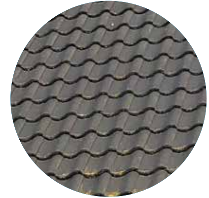
Black glazed pantile roof
