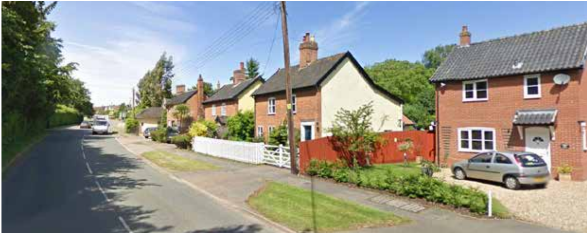
Figure 86: Two-storey detached and semi-detached houses along Lion Road, Palgrave.
