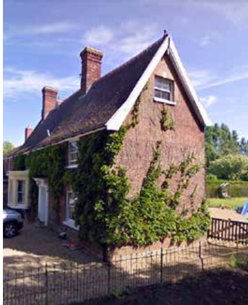
Figure 120: Stuston Place, the farmhouse associated with Place Farm.
