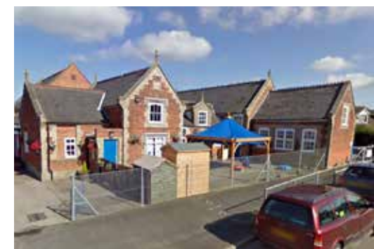
Figure 13: Primary School on Norwich Road.
