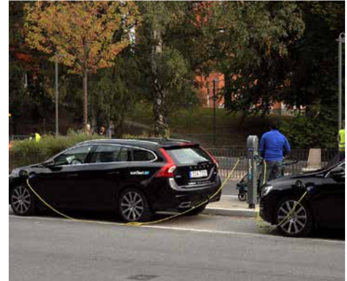
Figure 71: Inset parking with electric vehicle charging points.
