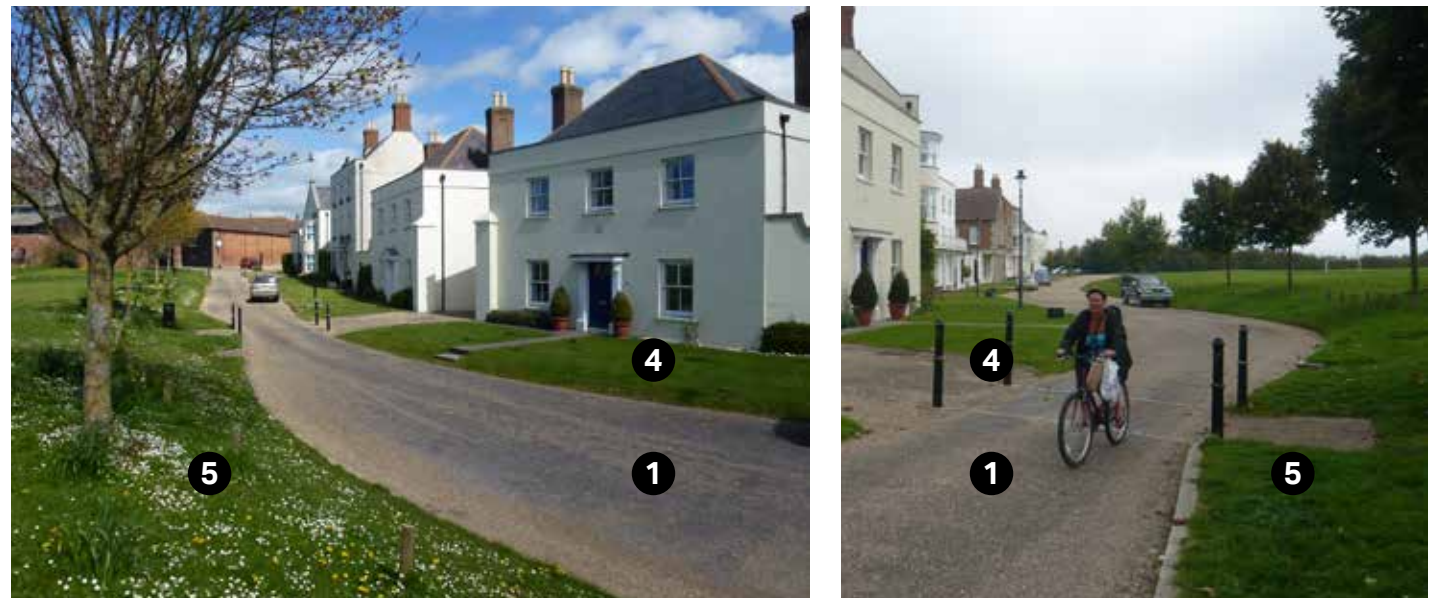
Figure 57: Examples of edge lanes in Dorchester, with low-speed roads shared between motor vehicles and cyclists, and opportunities for on-street parking (note: some localities may prefer clearly defined footways and parking bays).
