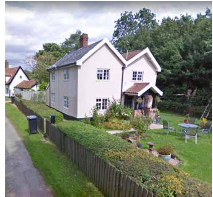
Figure 109: Building detail on Hall Lane, Shimpling.
