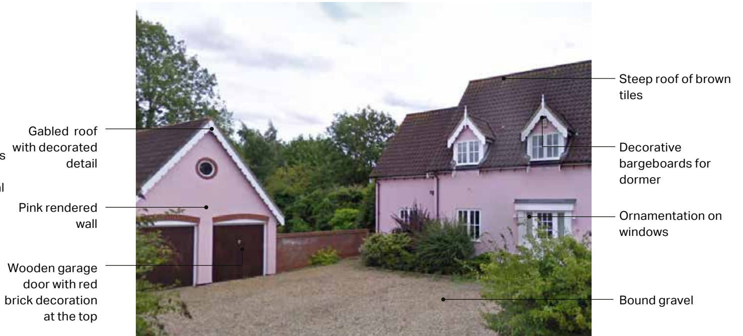
Figure 124: Architectural detail of a rendered building with on-plot garages on Talbots Meadow.
