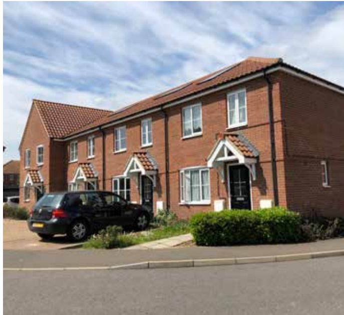
Figure 58: On-plot side parking on Spencer Crescent, Diss.
