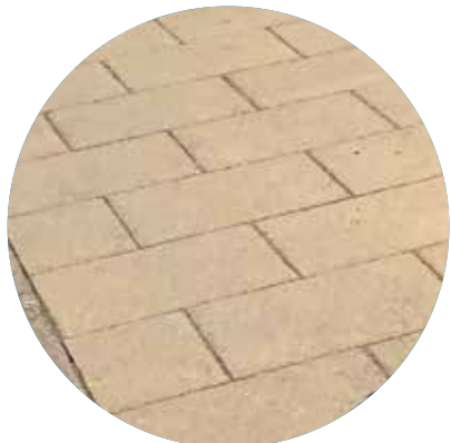
Yellow paving concrete
