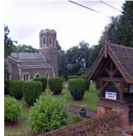
Figure 134: St Mary's Church on Rectory Road.
