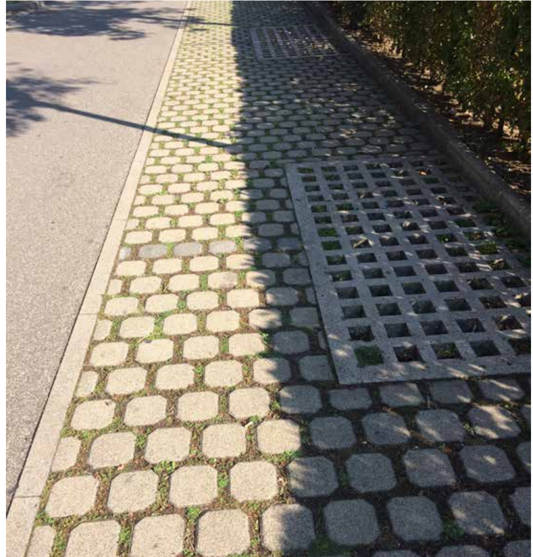
Figure 155: Example of permeable paving.
