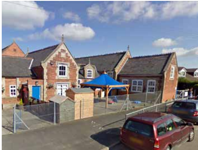
Figure 113: Primary School on Norwich Road.
