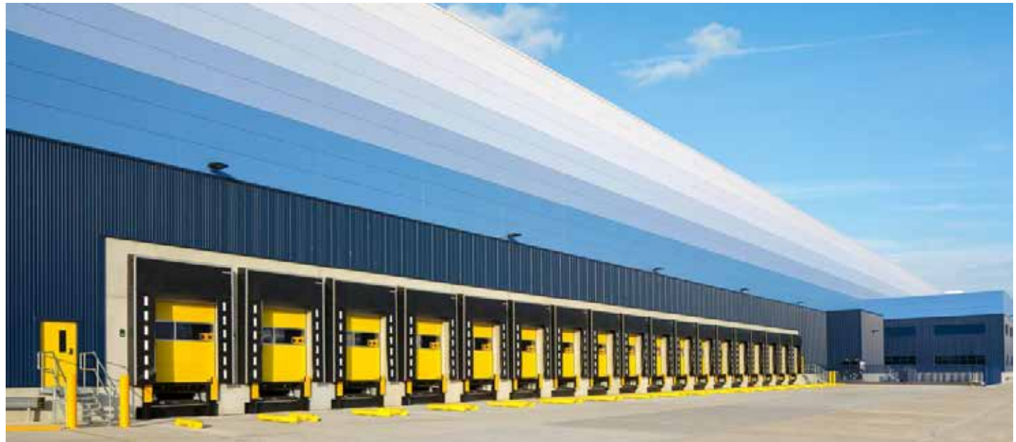
Figure 140: Large scale industrial park designed to disappear into landscape. Magna Park, Milton Keynes (Source: https://www.theguardian.com/artanddesign/2018/apr/15/shed-the-size-of-town-what-britains-giant-distribution-centres-tell-us-about-modern-life )
