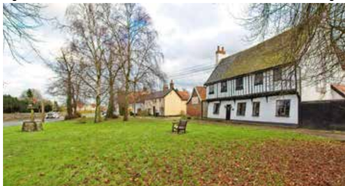
Figure 128: Exposed framing is unusual in Palgrave.
