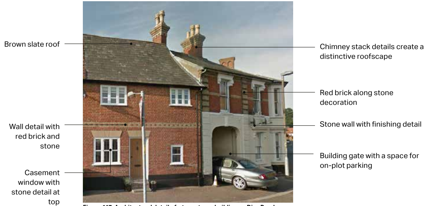
Figure 117: Architectural detail of a two-storey building on Diss Road
