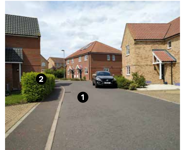
Figure 55: A shared lane in the north-east of Diss.
